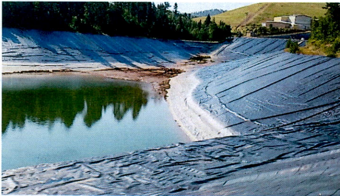
Storm water containment pond, water treatment plant in background (view from embankment)
