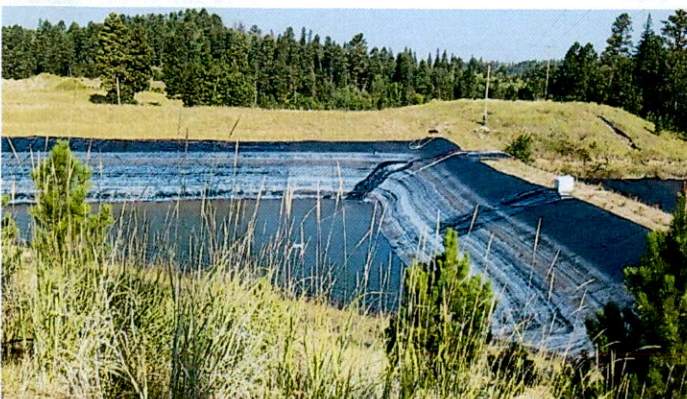
Feed Pond for water treatment plant
