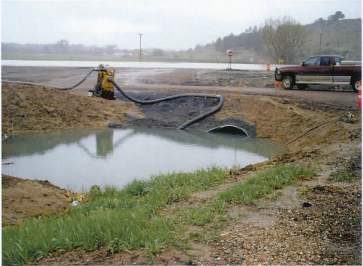
Looking in a westerly direction with the culvert in view
