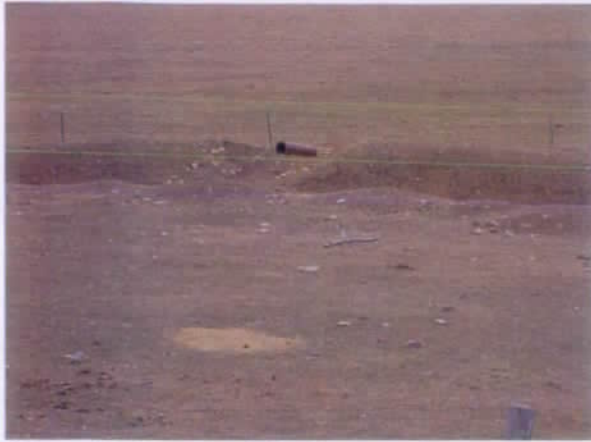
Photo #3 Breached ditch, no indication of recent use.
