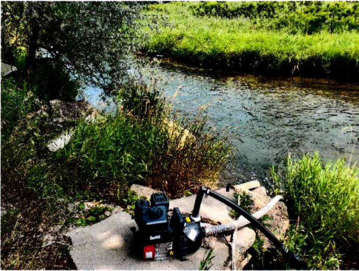
Centrifugal Pump at Redwater River diversion
