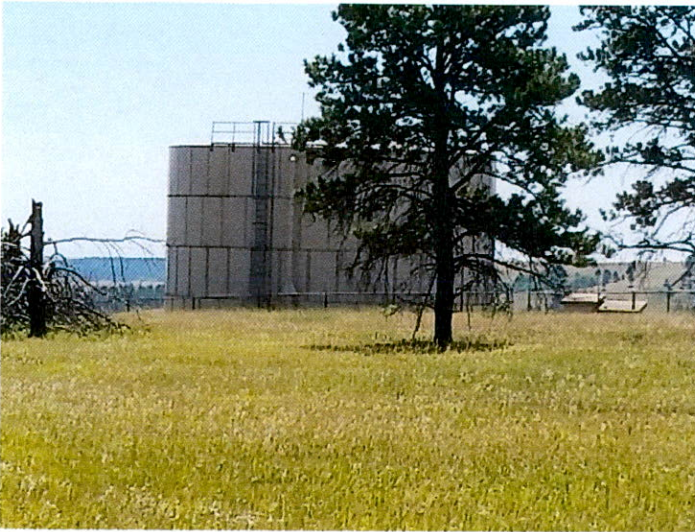
Fort Meade raw water storage
