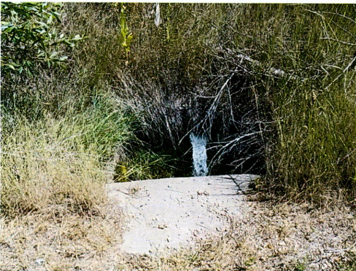
overflow outleting above service road and then into Bear Butte Creek
