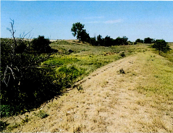
diversion on north side draw (SW \frac{1}{4} NW \frac{1}{4} S18) diversion dam in background
