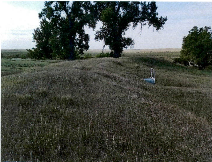
diversion dam (NW \frac{1}{4} NE \frac{1}{4} S13)
