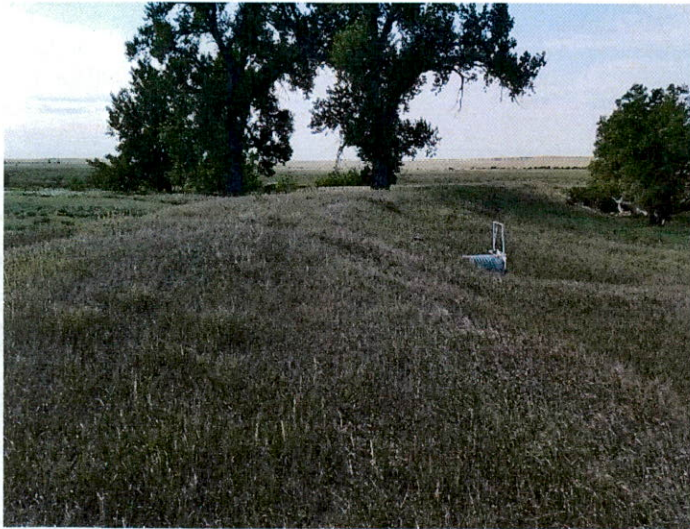
diversion dam (NW \frac{1}{4} NE \frac{1}{4} S13)
