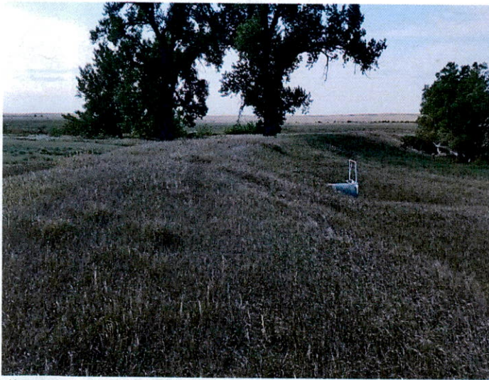
diversion dam (NW \frac{1}{4} NE \frac{1}{4} S13)
