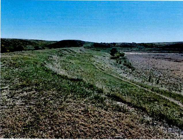
crest of large dam, pool area to right
