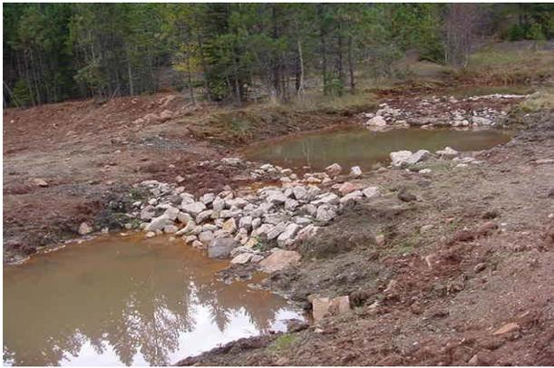
Photo 1.4 - Passive Treatment Ponds at Minnesota Ridge.
