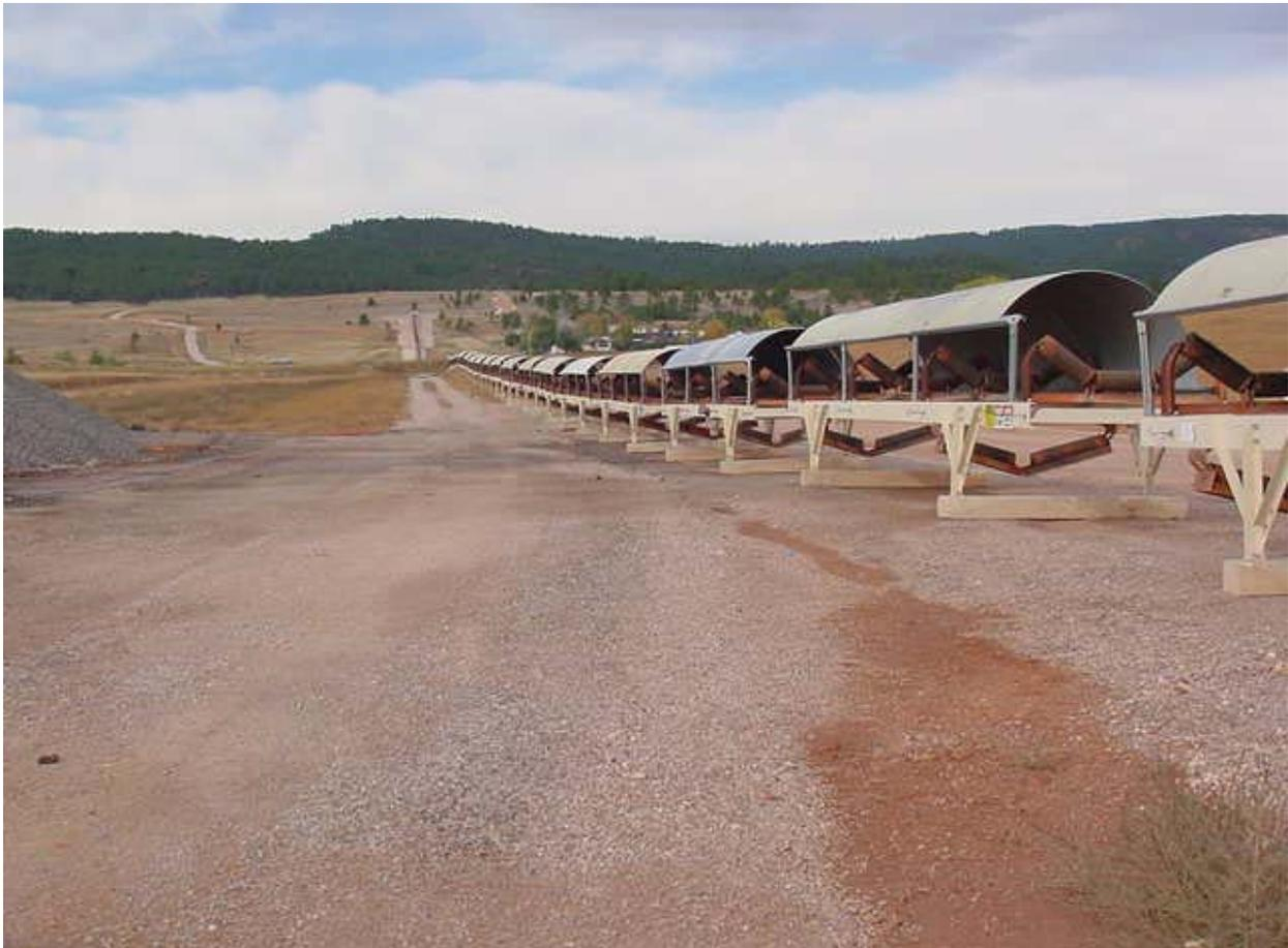
Photo 2.1 – Pete Lien and Sons Inc. installing conveyor in preparation for new Blackhawk Quarry northwest of Rapid City.
