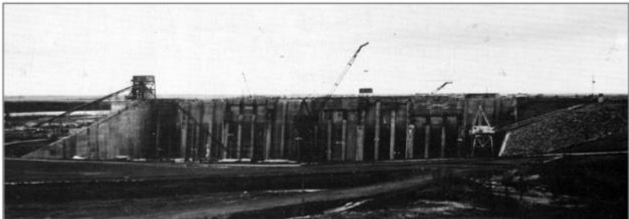
Figure 8-1. Diagrammatic view of Big Bend Dam area and photo of the Big Bend powerplant intake structure in final stages of construction prior to inundation.
