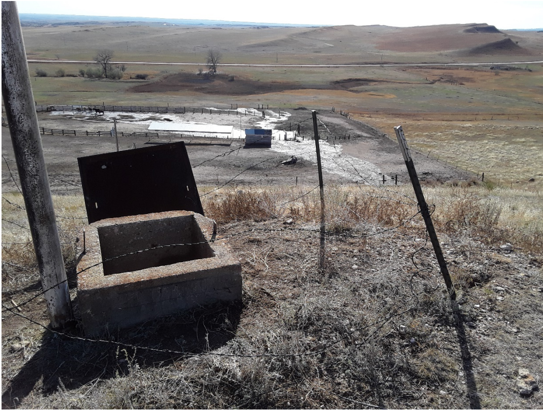
Access Hatch – No Weather Stripping Noted
