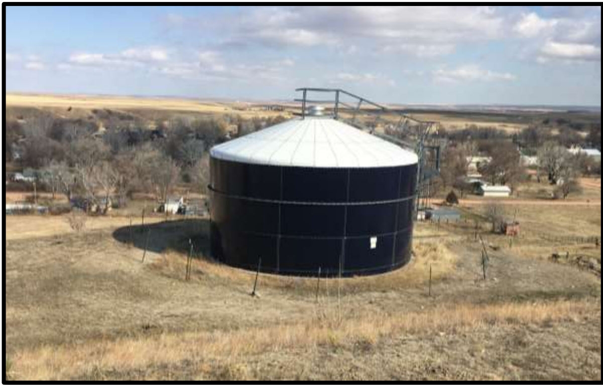
Figure 3.5-1: Ground Storage Tank Overlooking Town
