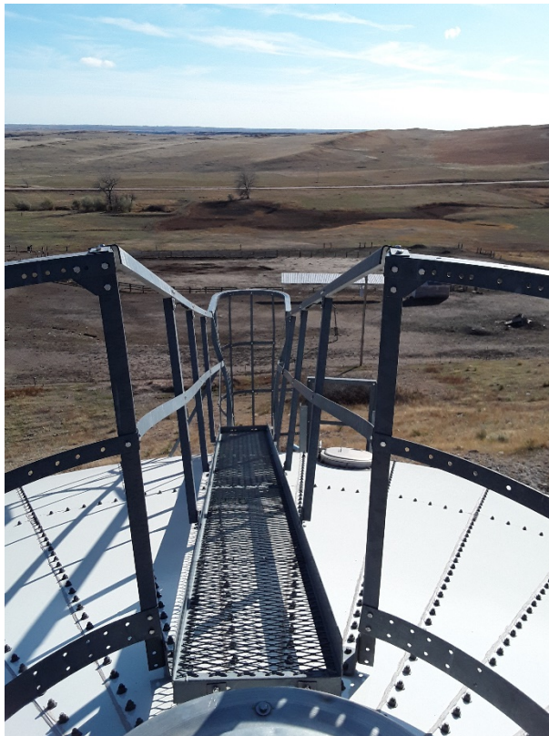
Exterior Ladder and Safety Rail
