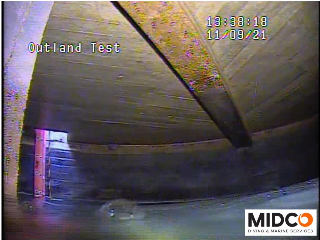
Wall to Roof Seam
