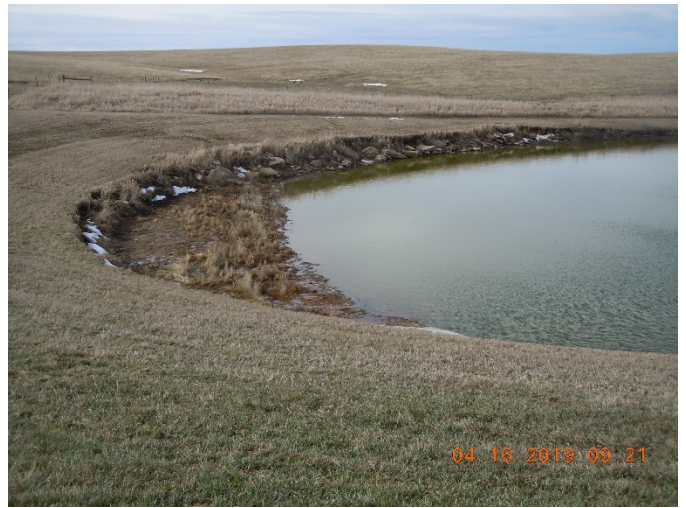
Figure 14: Seepage from Stormwater Pond to Cell #5
