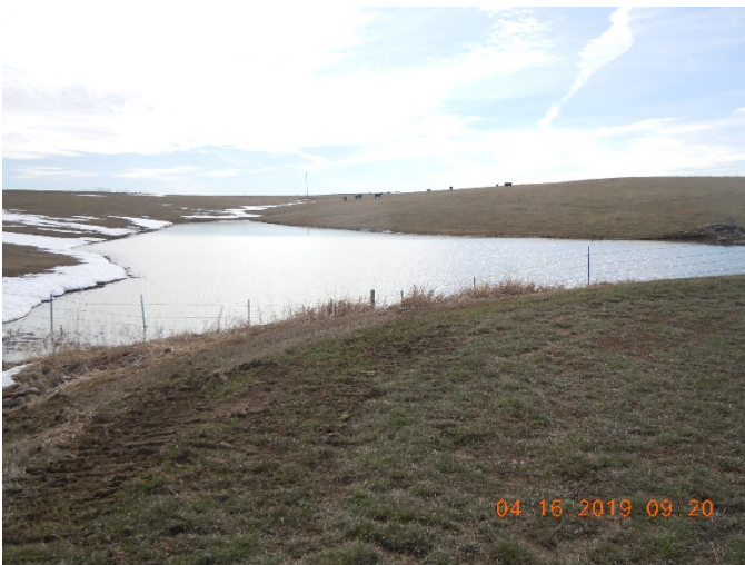
Figure 13: Stormwater Detention Pond
