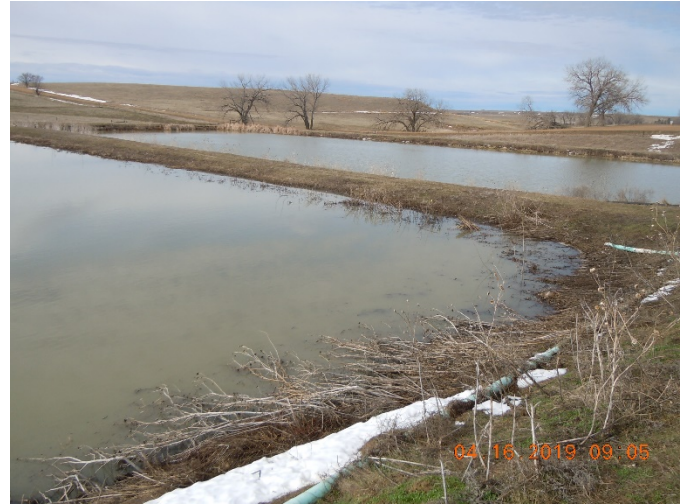
Figure 3: Cell #3 Facing Southwest
