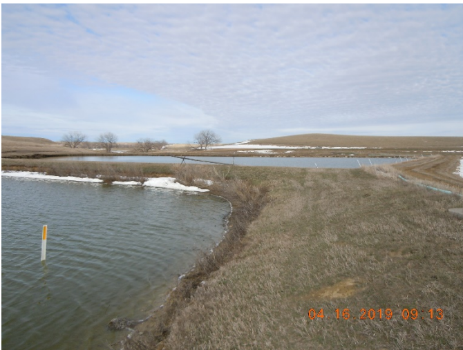
Figure 12: Cell #5 Facing West
