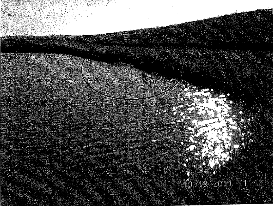
Photograph #1, erosion from overland flow into cell #4 is circled.
