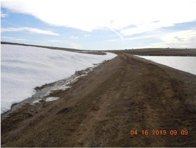
Figure 5: Storm Water Canal Facing East
