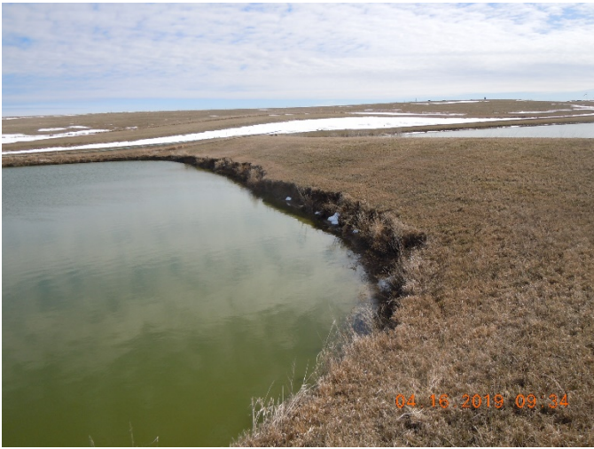
Figure 18: Erosion on Cell #4
