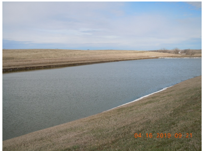
Figure 15: Cell #5 Facing Southwest
