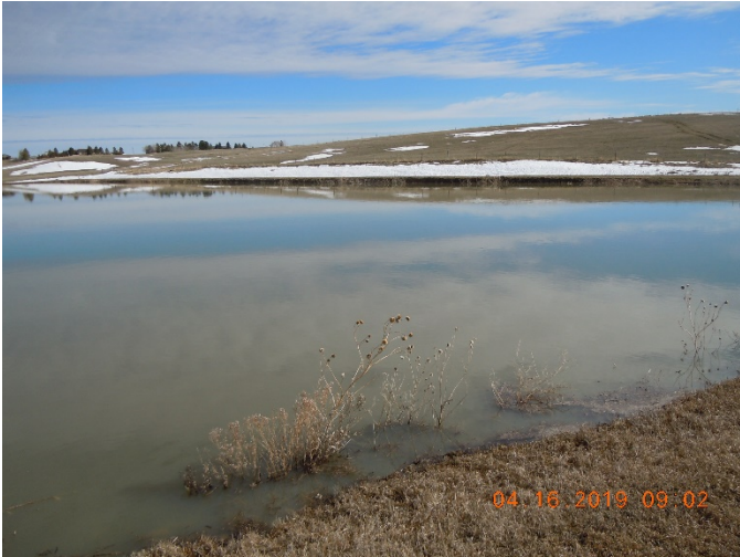
Figure 1: Cell #1 Facing North
