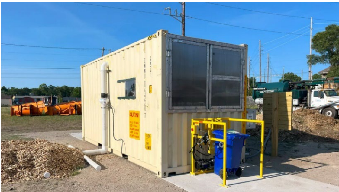
Figure 3-1: Traverse City In-Vessel Composting System
