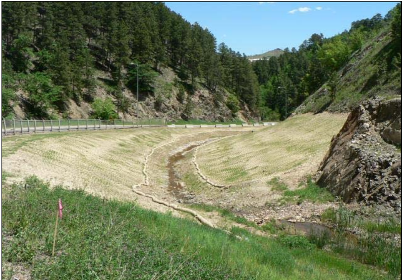
Photo 1.4 – Reclaimed portion of Gold Run Creek after removal of Homestake’s Slurry Plant.
