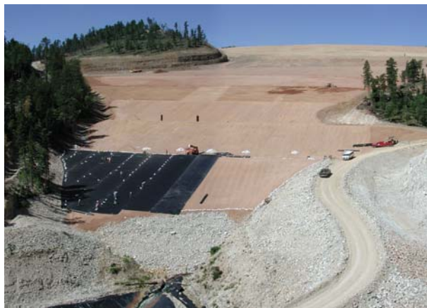
Photo 1.3- Liner Placement on Ruby Dump.
