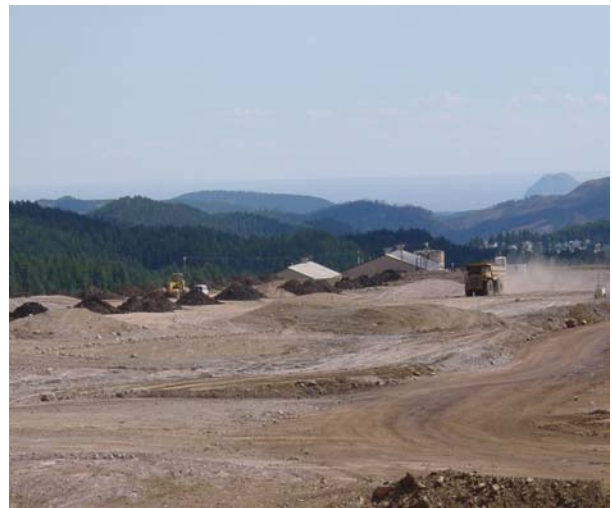
Photo 1.6 – Reclamation work on leach pad.
