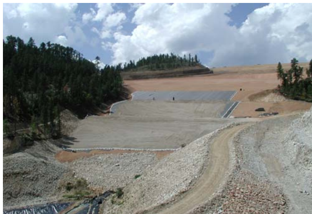
Photo 1.4 – Drain layer placed on top of liner.
