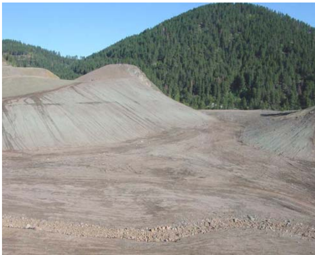
Photo 1.5 – Backfilled and recontoured East Liberty Pit
