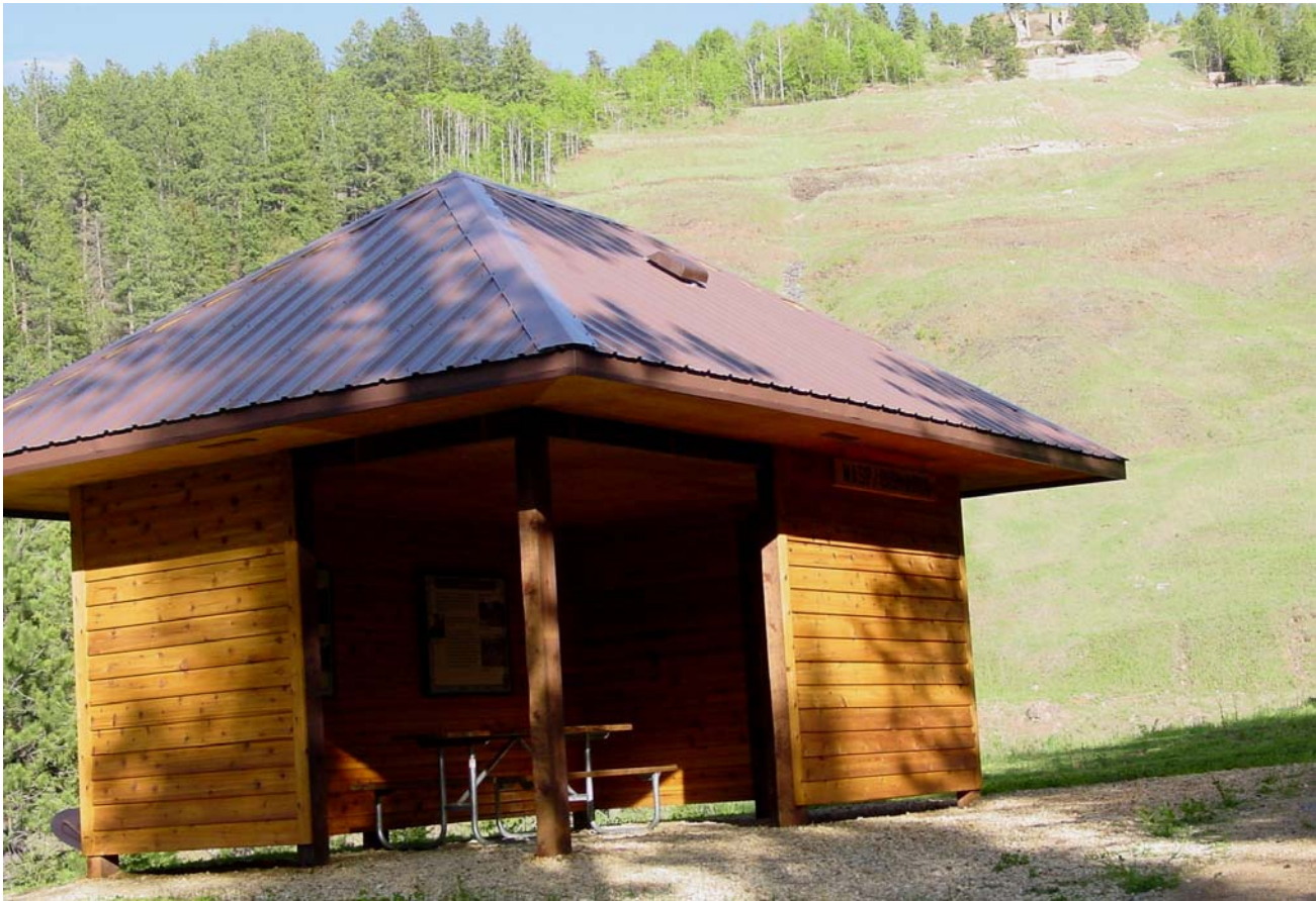
Photo 1.1 – Visitor Center constructed by Homestake Mining Company at reclaimed Wasp Tailings on Whitewood Creek south of Lead.
