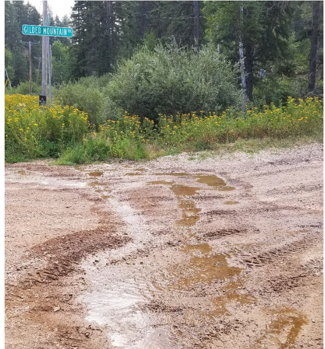
Photo 4-8: Road intersection immediately upstream of Site FC-1-BIO likely acting as a source of sediment to the stream, August 2020.
