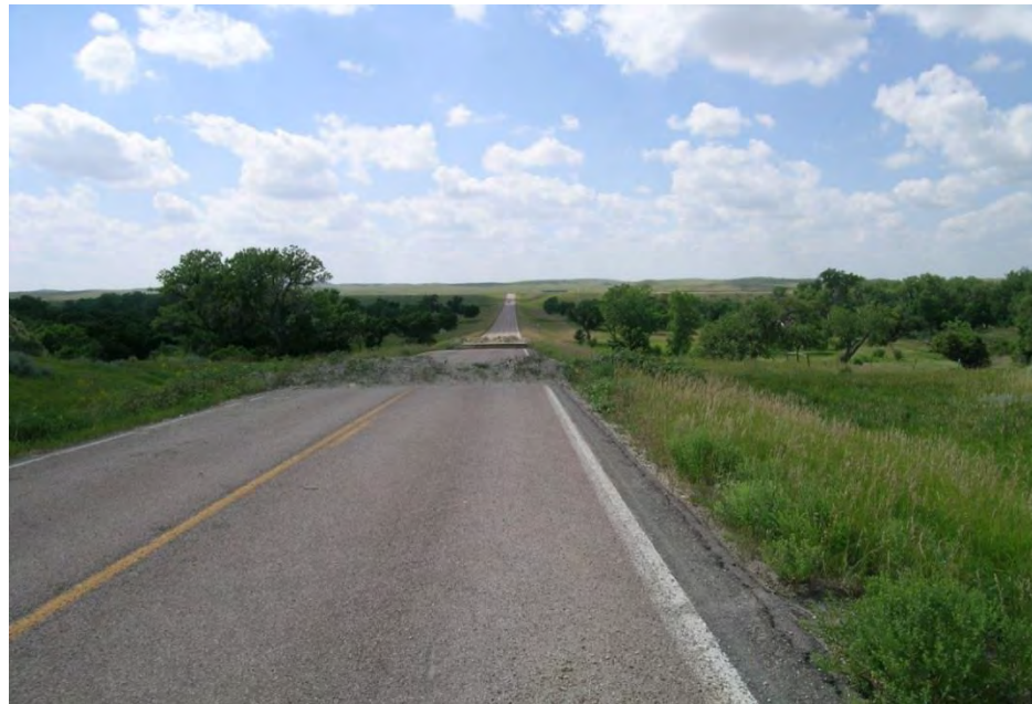
Figure C-4. Site 4, on the White River, west of Pine Ridge, SD, BIA Highway 32, 2011. The culvert washed out the road at the site in a flash flood.
