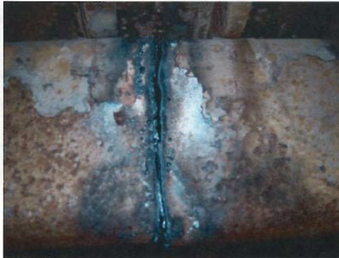
Photo #4: Chassis rail cut in half
