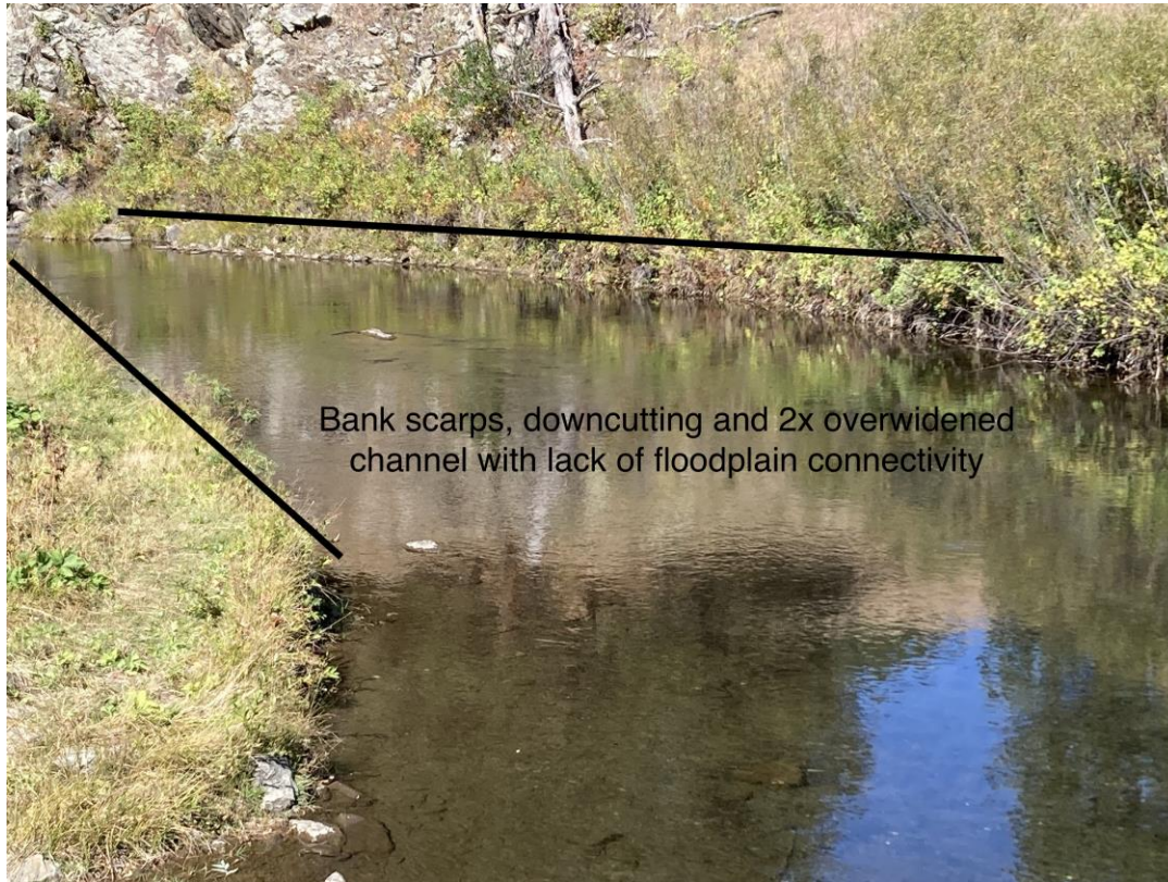
Figure B3. Photo showing bank scarp evidence of channel downcutting and past erosion with 2x overwidened channel from expected dimensions.
