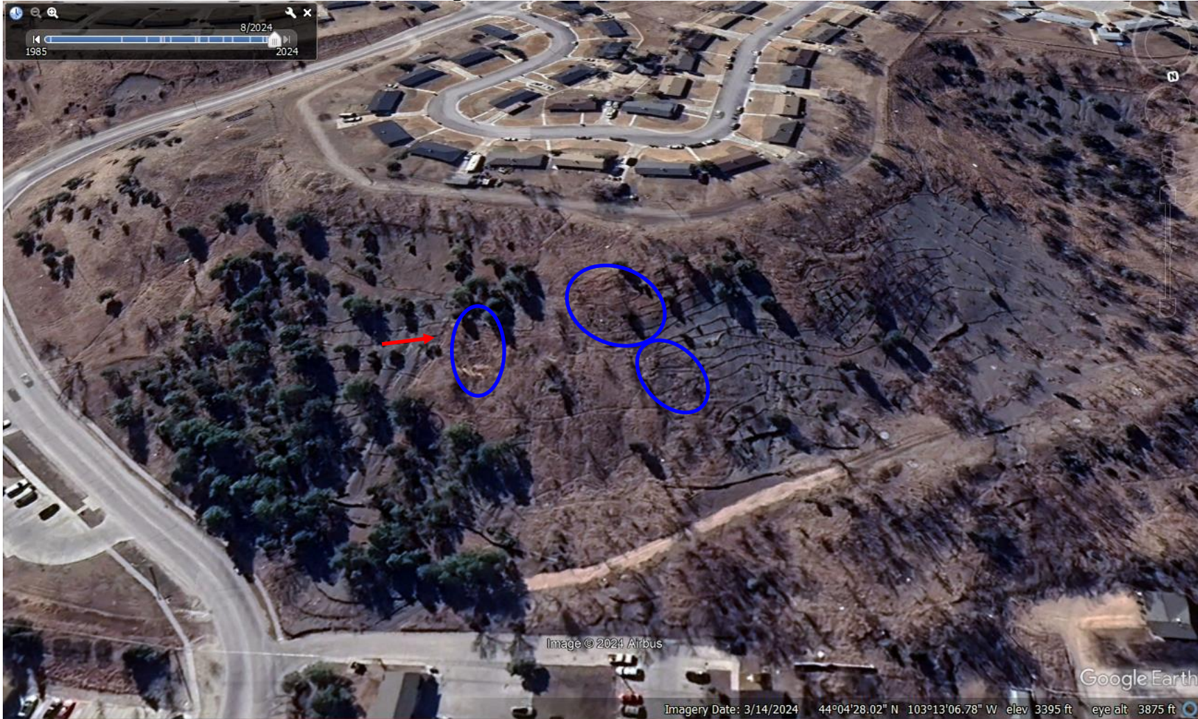
Figure A4. Google Earth image (March 14, 2024) showing Star Village project site after continued implementation. Red arrow shows location of treated side cut shown in figure 7. Blue ovals show partially eroded areas that have been treated with yard waste. Red arrow shows location of a side cut that is shown in figure 7.
