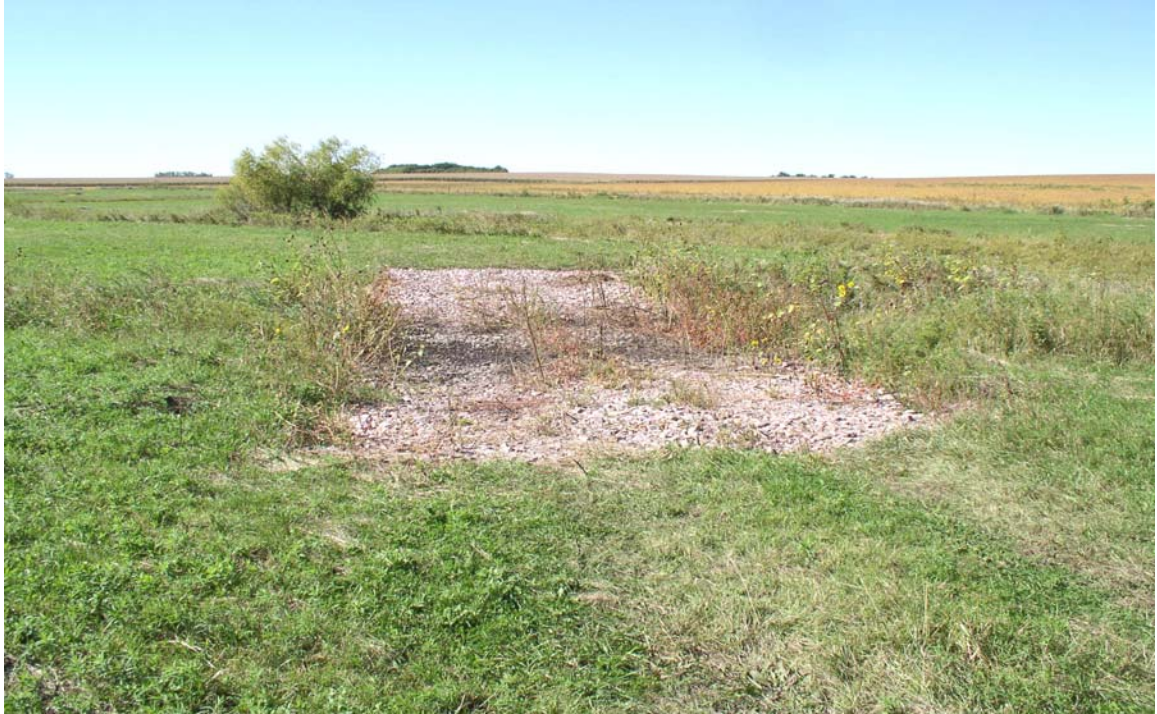
Rock Crossing Installed to Reduce Bank Erosion (Bachelor Creek HU Project).
