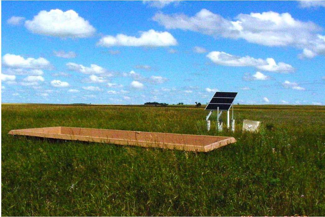
Solar Powered Well and Stock Watering Tank Installed to Provide an Alternate Water Source for a Managed Grazing System (Blue Dog Lake Watershed Project).
