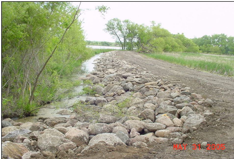
Bourne Slough Berm Stabilized Using Riprap (Herman/Madison/Brant Watershed).
