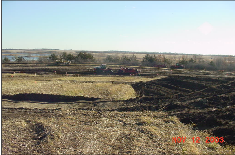
Excavation of Evaporation Pond for Animal Nutrient Management System (Herman/Madison/Brant Watershed).
