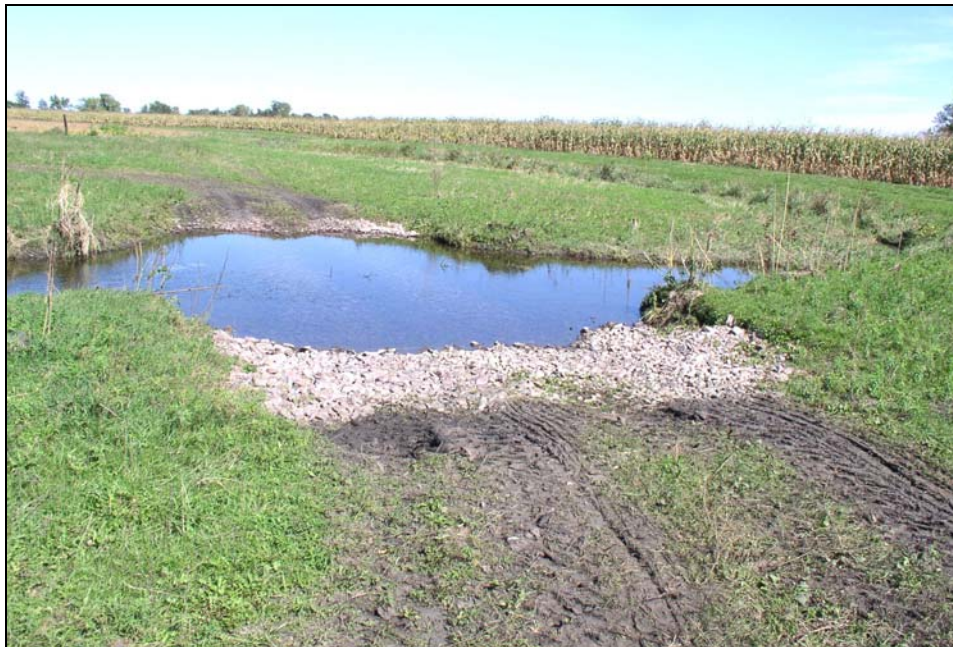
Rock Crossing Installed to Reduce Bank Erosion (Bachelor Creek Watershed).
