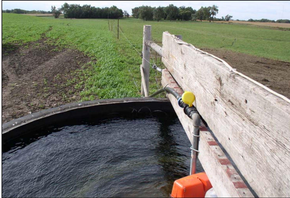
Alternative Water Source Using a Tank Supplied With Water From a Rural Water System Using Above Ground Pipeline (Bachelor Creek Watershed).
