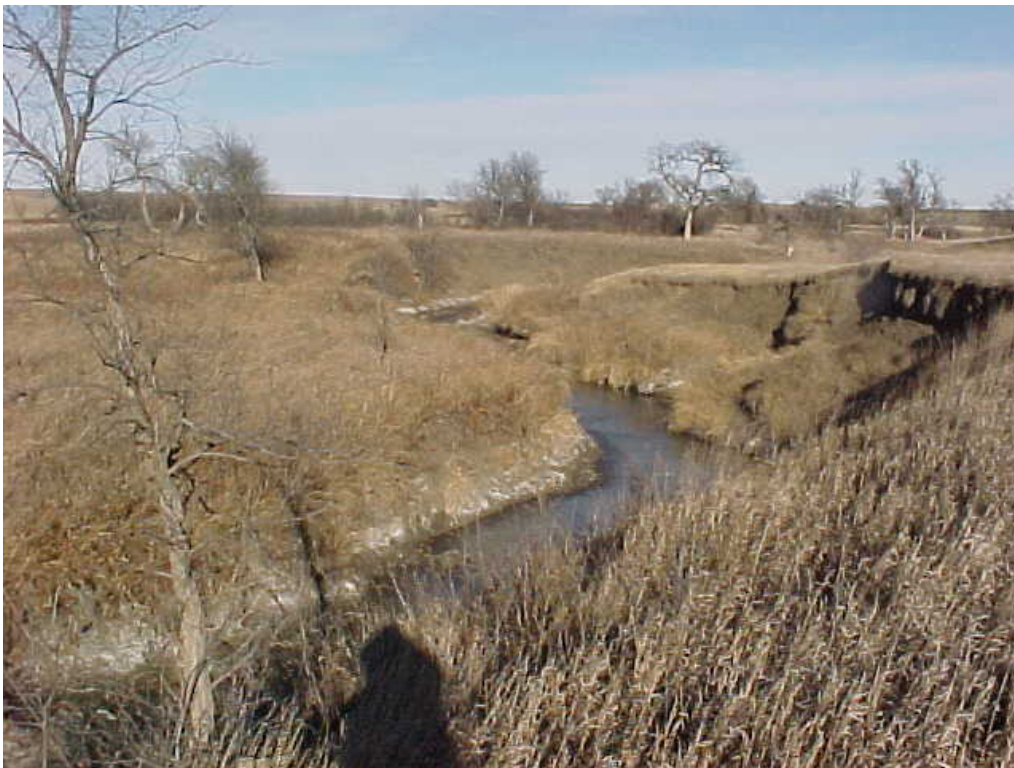
Figure 20. Mainstem Medicine Creek showing bank failures and widening between Presho and Kennebec, Lyman County, South Dakota in 2004.
