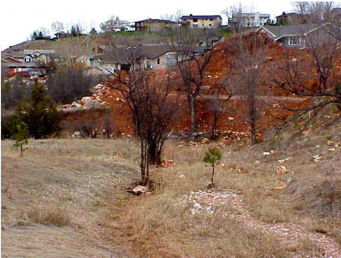
Figure 3: This photo shows how a contractor has placed construction debris along a cutbank in the Wonderland drainage channel.
