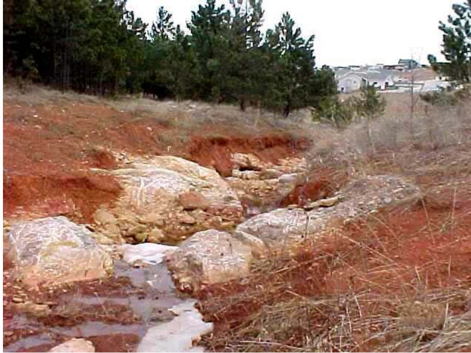
Figure 9 - Incision and Widening of the Main Drainage Channel
