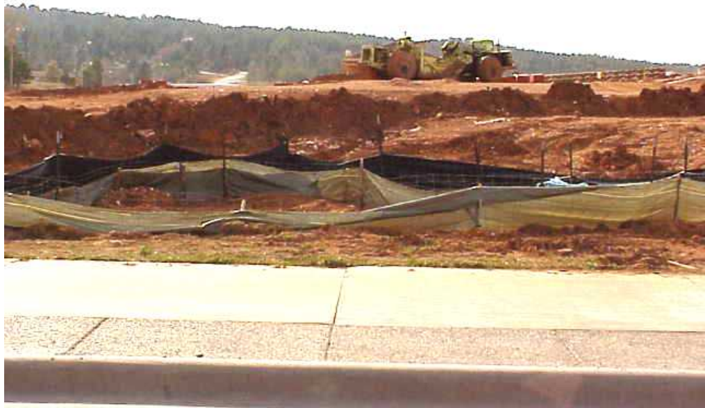
Figure 1: This photograph shows a poorly constructed silt fence with an “earthen dam” placed behind it to control the stormwater runoff.
