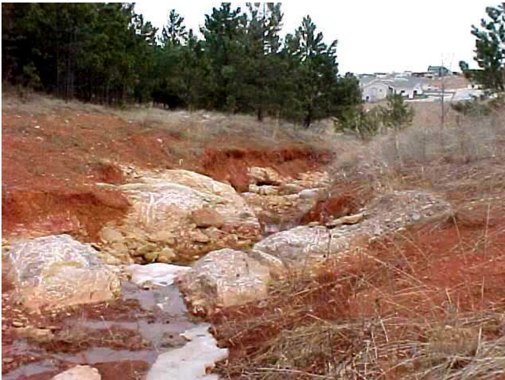
Figure 4: Recent development above this section of the Wonderland drainage channel has increased the stormwater runoff within the basin. This increase in runoff has eroded the channel significantly the past two years. This photo shows how the channel has been eroded down to the bedrock.
