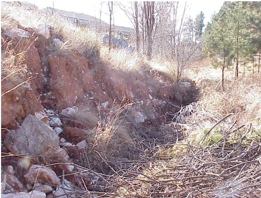
Figure 3.3 Bank erosion of fill material placed for earlier development.
