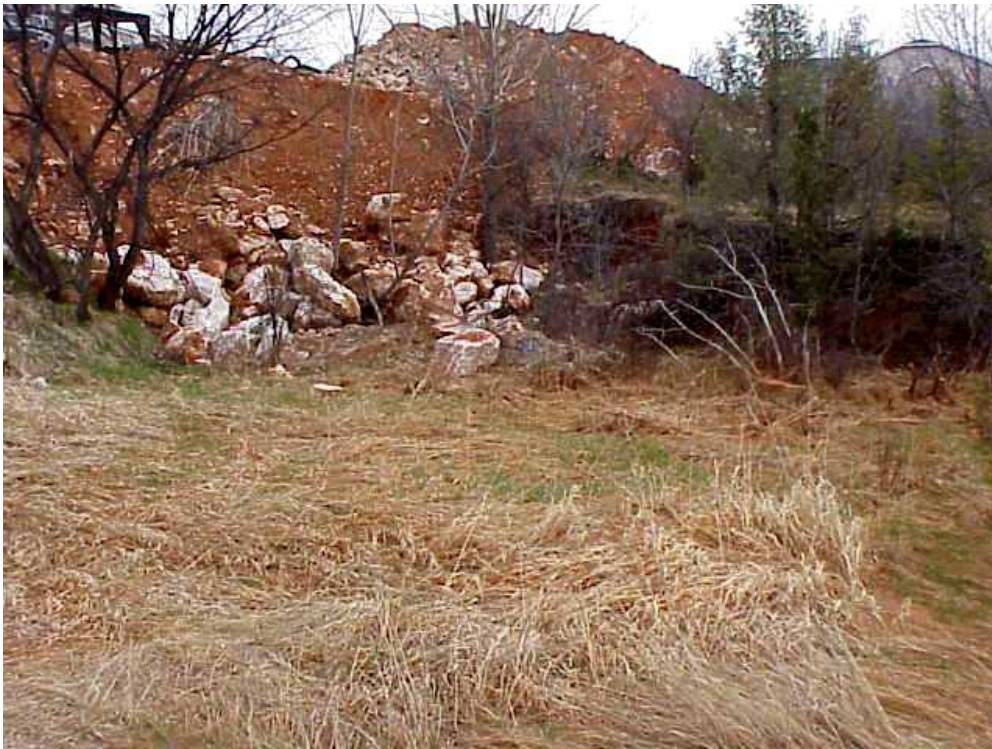
Figure 5: Recent construction within the Wonderland drainage basin will not only increase the flows within the channel due to an increase in imperviousness, but, as can be seen in this photograph, poor construction practices have also led to debris being placed directly into the channel. This construction debris will ultimately degrade the water quality within Wonderland drainage basin and Rapid Creek.
