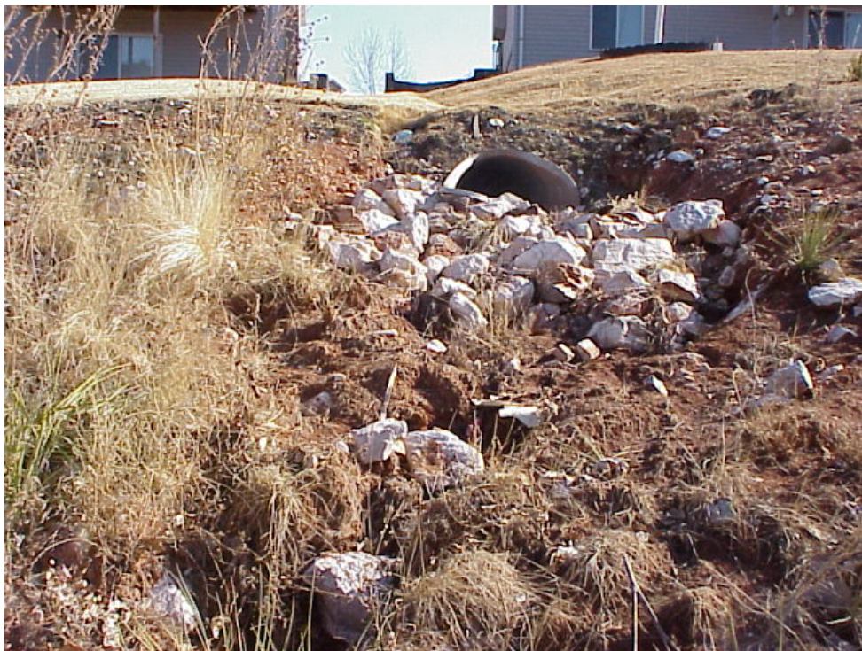
Figure 3.5 Outlet of storm drain with inadequate erosion control. Outflow directed to very steep bank.
