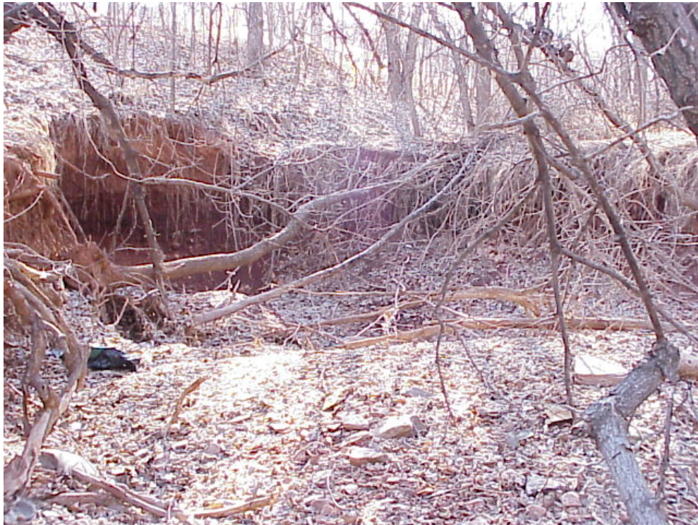
Figure 3.1 Photograph looking upstream at head cut in Wonderland Basin main drainage channel.
