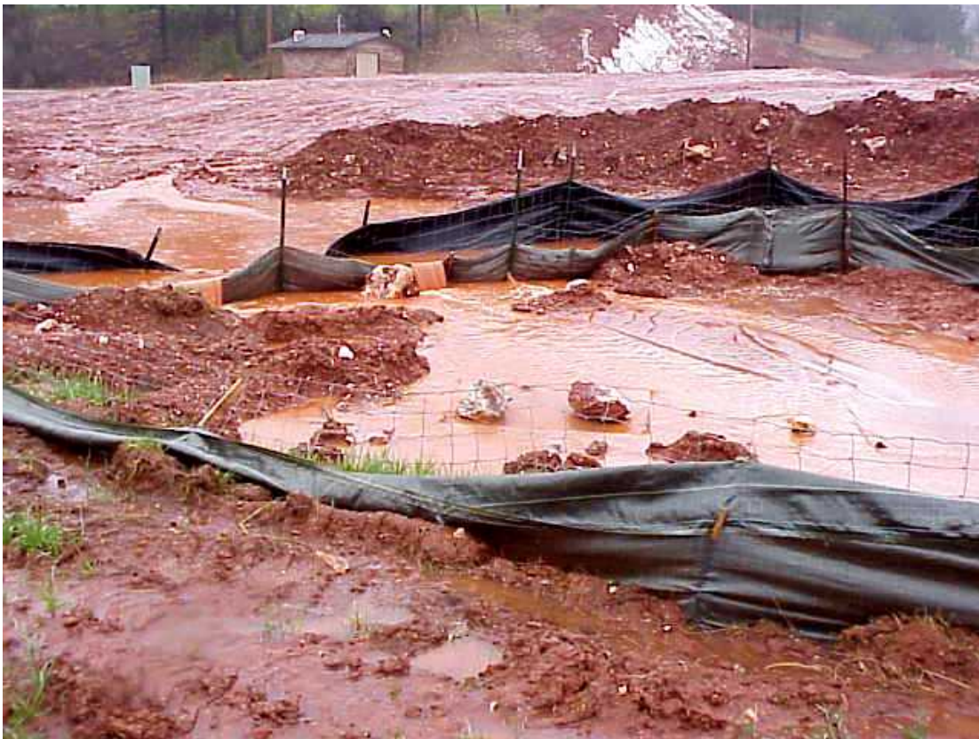
Figure 4: Stormwater pollution from this site in the Arrowhead drainage basin could have been prevented with properly constructed silt fences and detention facilities.
