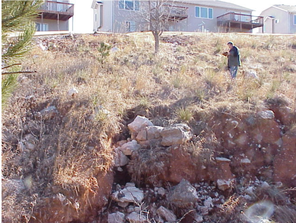
Figure 3.4 Intersection of storm drainage with main drainage. Storm sewer outlet directed over steep bank fill material.
