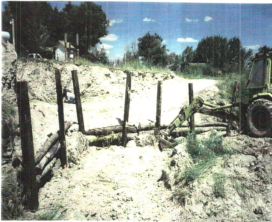
A stream bank stabilization structure under construction using log cable anchors and erosion fabric. When completed the structure was vegetated with native woody plants.
