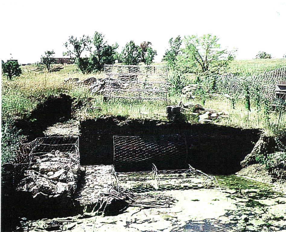
The structure designed used gabion baskets filled with rock to serve as a drop structure. The photograph above is of the structure while under construction.
