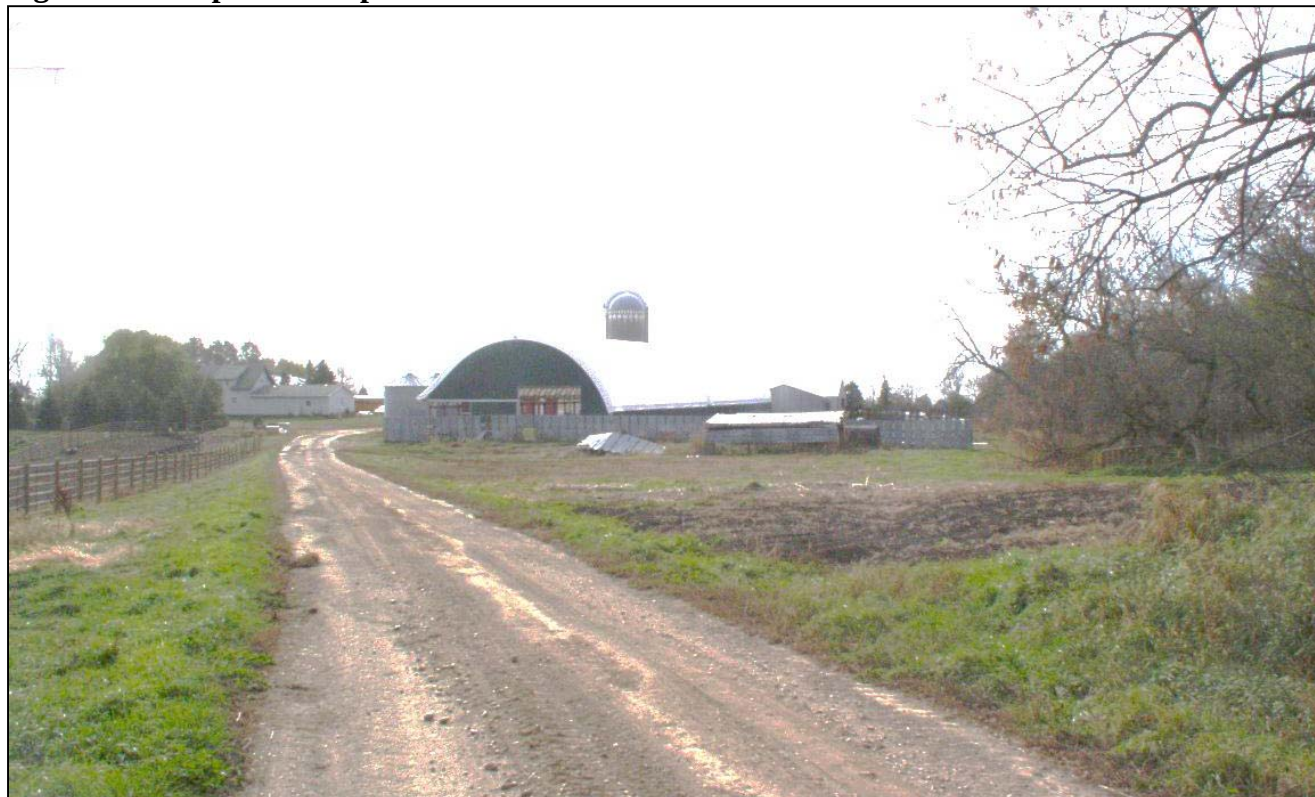
Figure 8: Completed Hoop Barn
