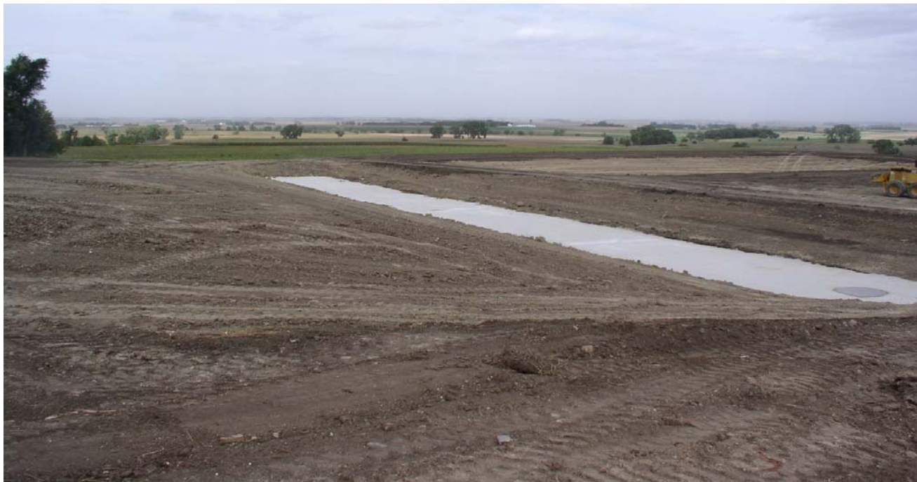
Figure 7: Completed Open Lot Sediment Basin and Pond
