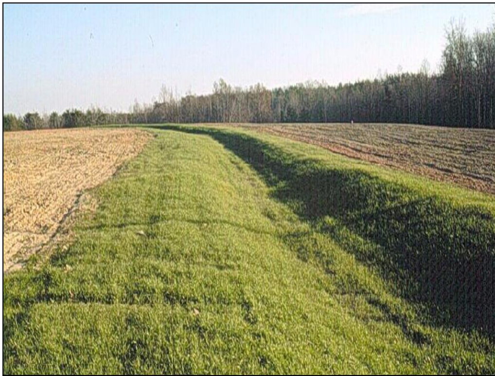
Figure 6. Filter strip installed to reduce NPS loading from cropland.
