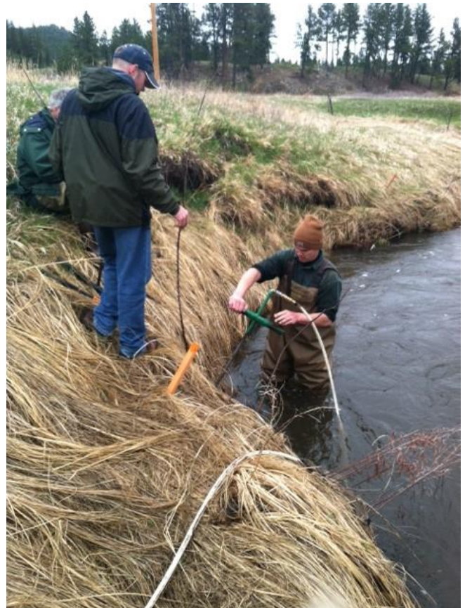
Figure 4. Willow Planting along Streambank
