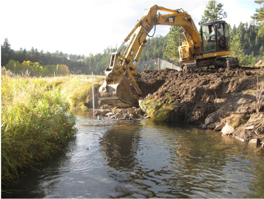
Figure 4-3. Riparian Buffer and Streambank Protection Best Management Practice Installation Along Spring Creek Near Hill City, South Dakota.
