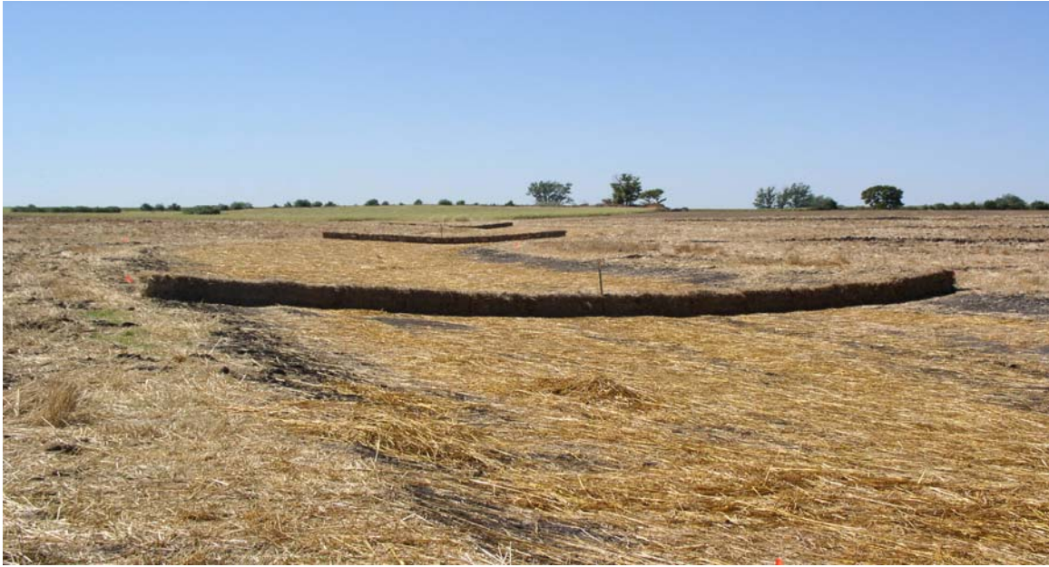
Figure 14. New waterway with erosion control in place.
