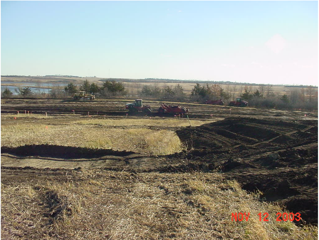
Figure 6. AWM System Six – Excavation of Evaporation Pond.
