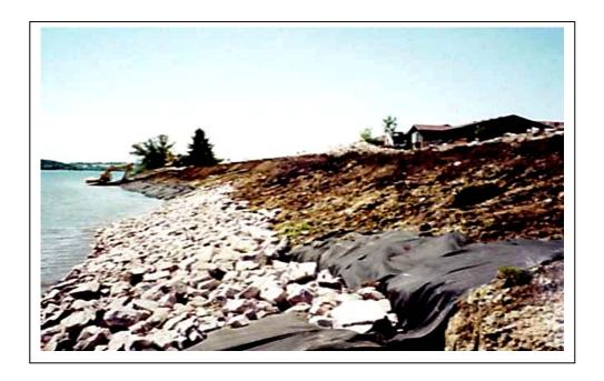
During the course of the Lake Hendricks project 1,575 linear feet of shoreline was stabilized with the use of filter fabric and granite quartzite rock riprap. This reduced shoreline erosion and sedimentation on three separate areas around Lake Hendricks.
