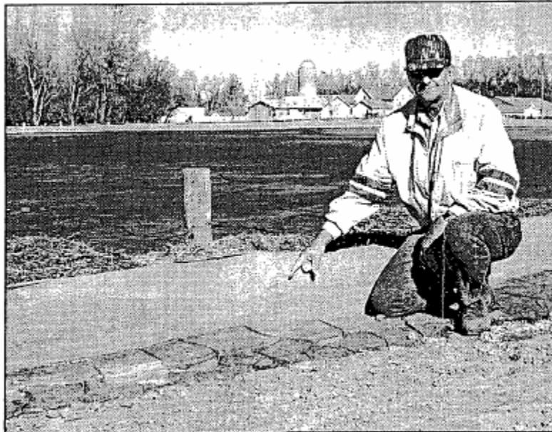
LeRoy Stohr, project manager, points to the top eight inches of one of the sediment ponds. Stohr is standing on over three feet of silt, which has already hardened in this holding area.
