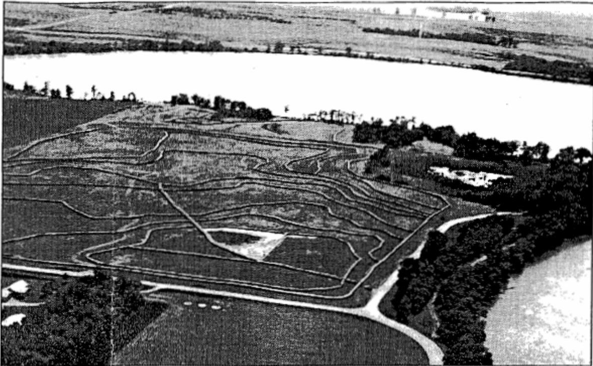
This picture shows the different ponds that have been set up on the land just east of the lake. Already six or more of these ponds have been filled or partially filled with sediment. The water will eventually return to the lake at the top of the photo after going through a series of holding ponds where the sediment will sink to the bottom.
