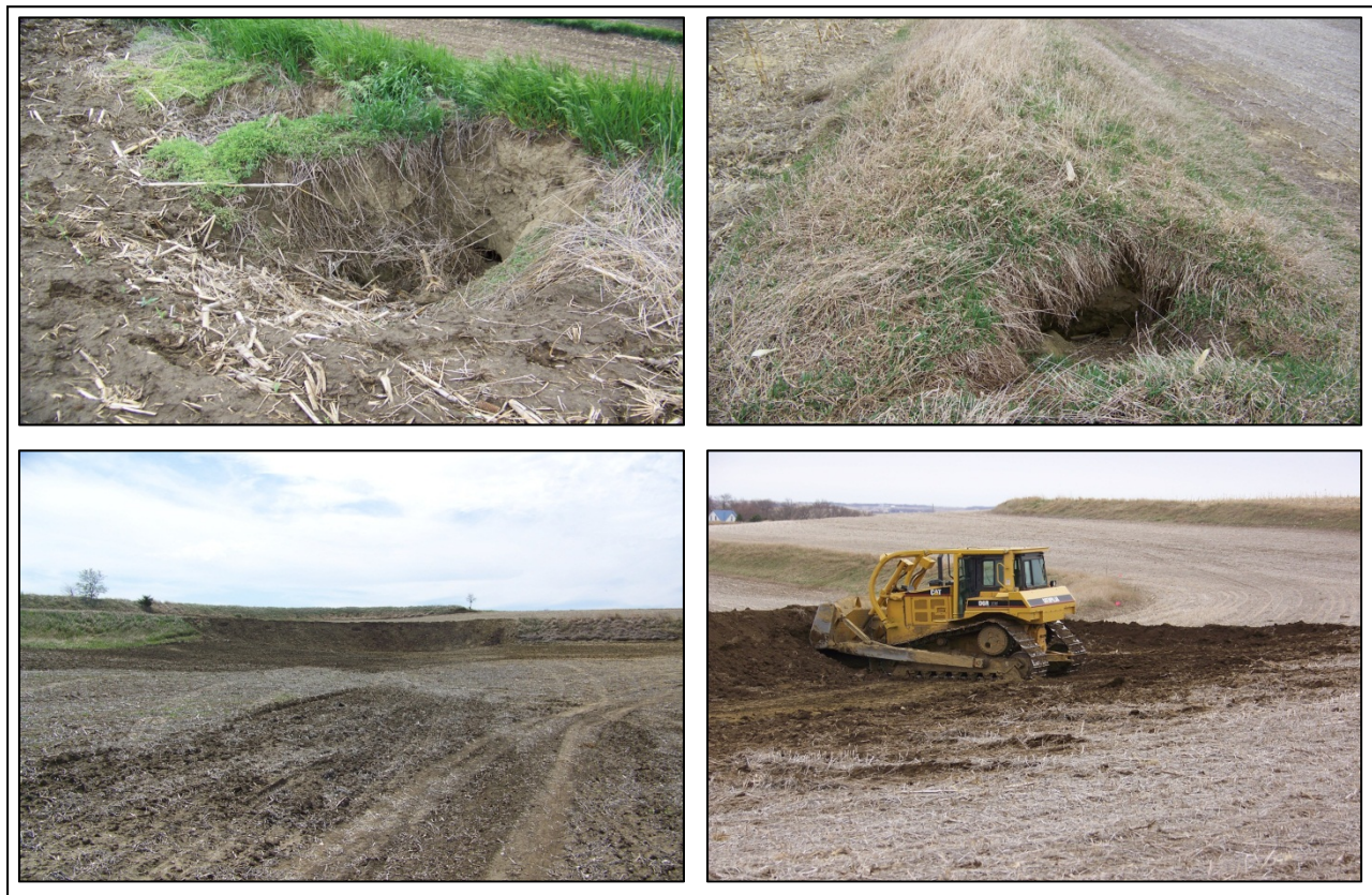
Figure 3: Terrace Restoration Project
