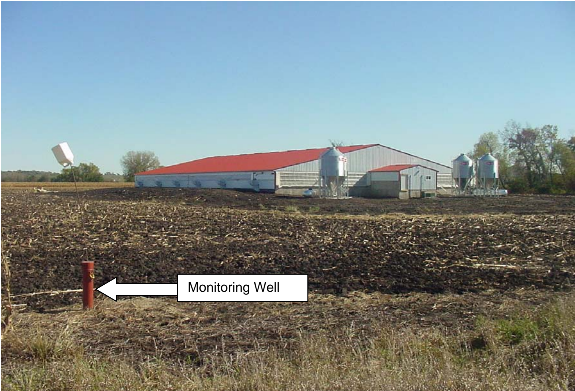
Figure 10: Completed 2,400 Head Hog Facility with Ground Water Monitoring Wells
