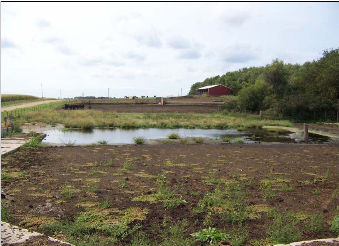
Figure 12: Feedlot VTA Established with Ponding Water
