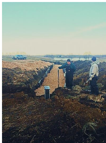
Figure 15: Bioreactor with Woodchips
