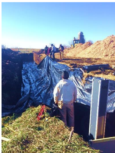
Figure 14: Bioreactor Lining
