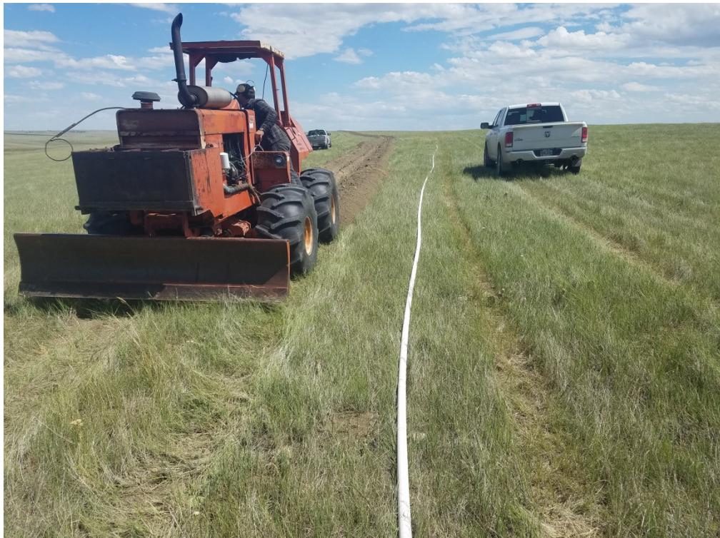
Figure 3-8. Livestock Water Pipeline Installation.
