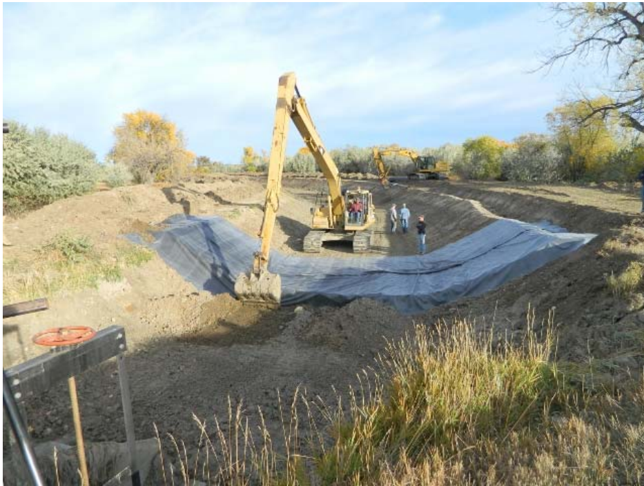
Figure 3-4. Lining the South Canal.
