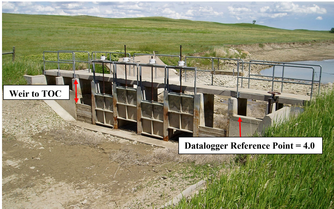
Figure 25. Illustration of weir to TOC measurement and the 4.0 reference point located at the top of the overflow weirs.
