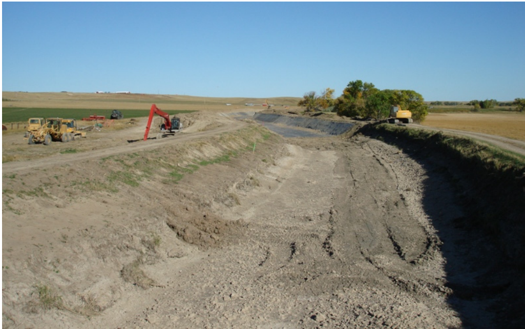
Figure 3-5. Lining of the Inlet Canal.
