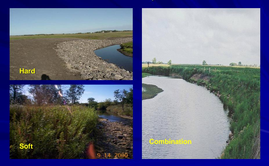
Use of plants and plant materials (brush) and engineered structures for slope protection and erosion control.
