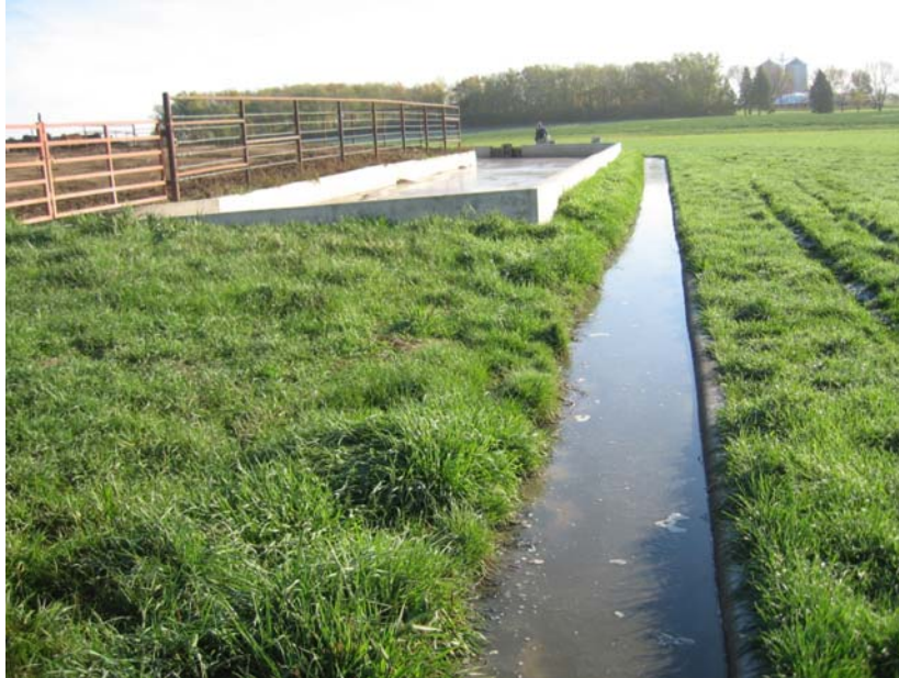
Figure 17. Side view of the Stevens VTS at the south end, looking ENE. In the image are pens (far left), sediment basin (within the concrete walls), curb-and-gutter distribution system (center of image), and the VTA (far right). Runoff flows from left to right in the image.
