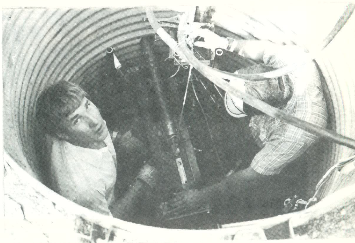
Figure 3-5. Using the lateral drilling machine to make a hole 6' away from the manhole wall for installation of the porous stainless steel cylinder.
