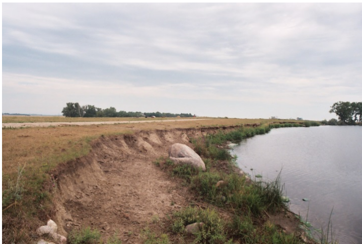
Figure 5. Amsden Dam before Stabilization
