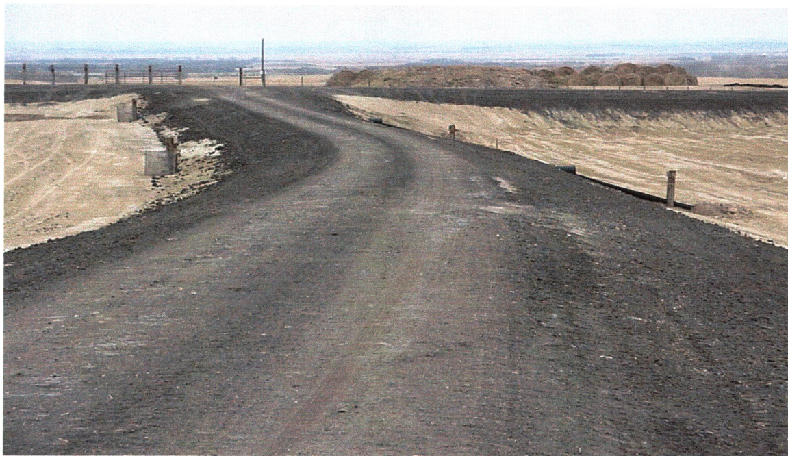
The animal waste management system constructed for Frank Rinas. The sediment basin with screened inlets is on the left, and the evaporation pond is on the right.
