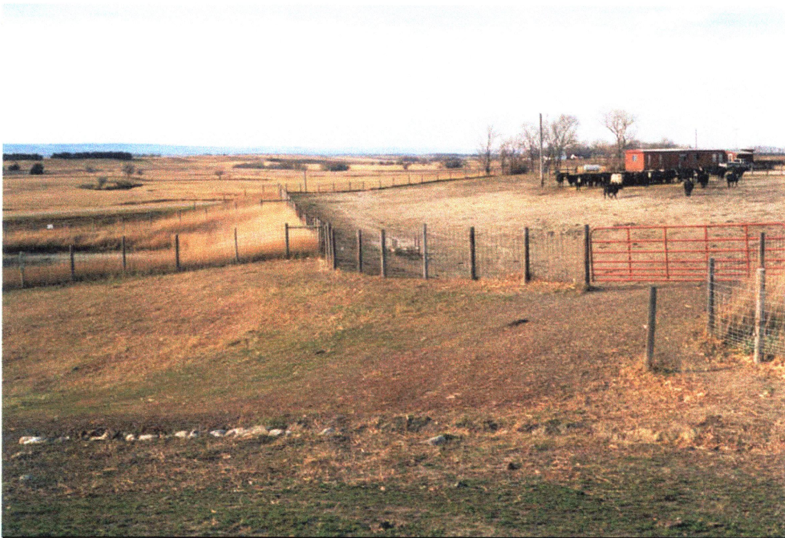
An animal waste system built for Scott Nelson in 1998: holding pond to the left, sediment basin to the right.
