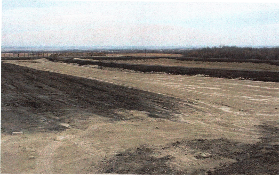
An animal waste management system was constructed for Frank Rinas in the fall of 1999. The sediment basin is in the foreground, and the evaporation pond is in the background.
