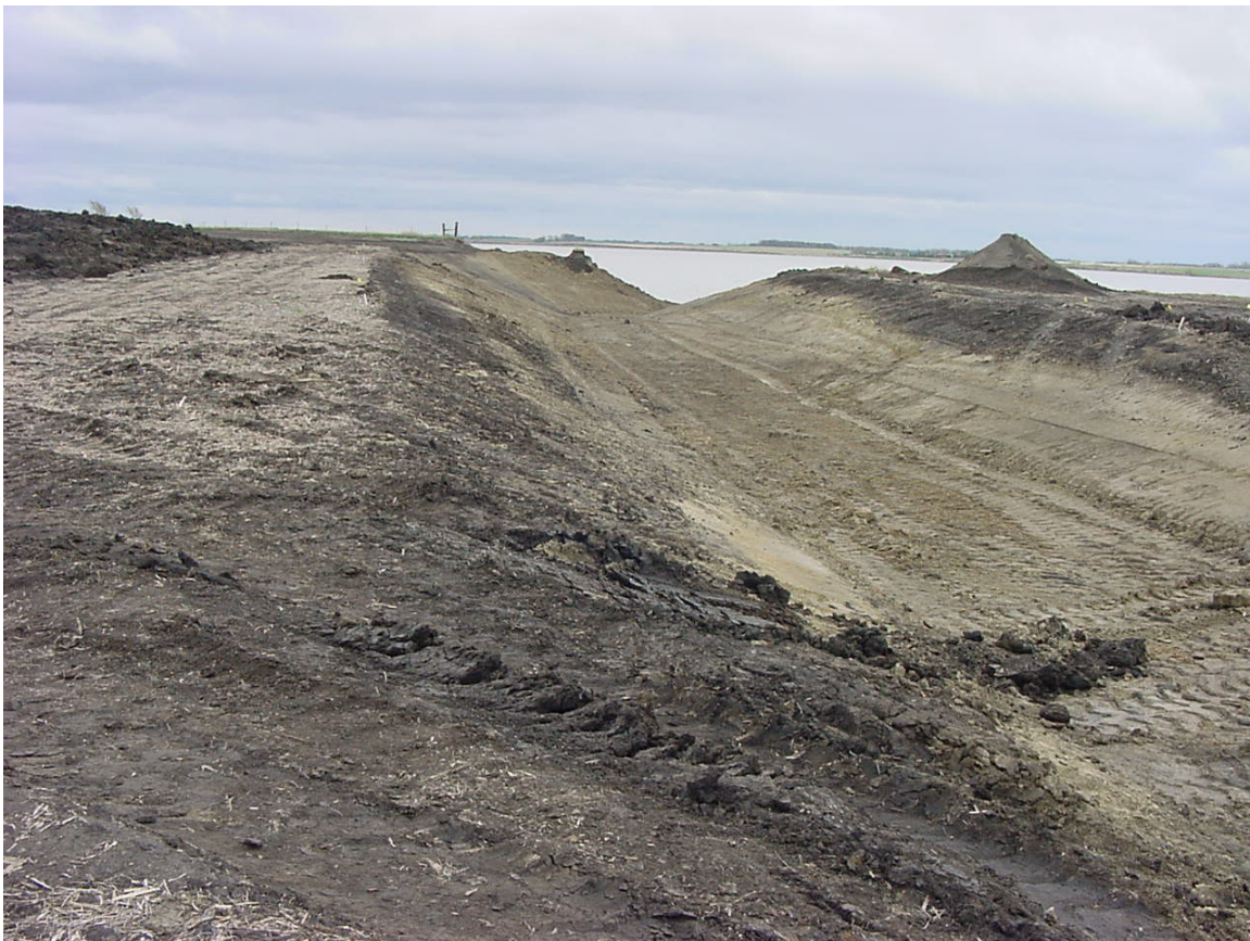
Figure 20. Clean water diversion that was being built in conjunction with the animal waste management system for feedlot number 11
