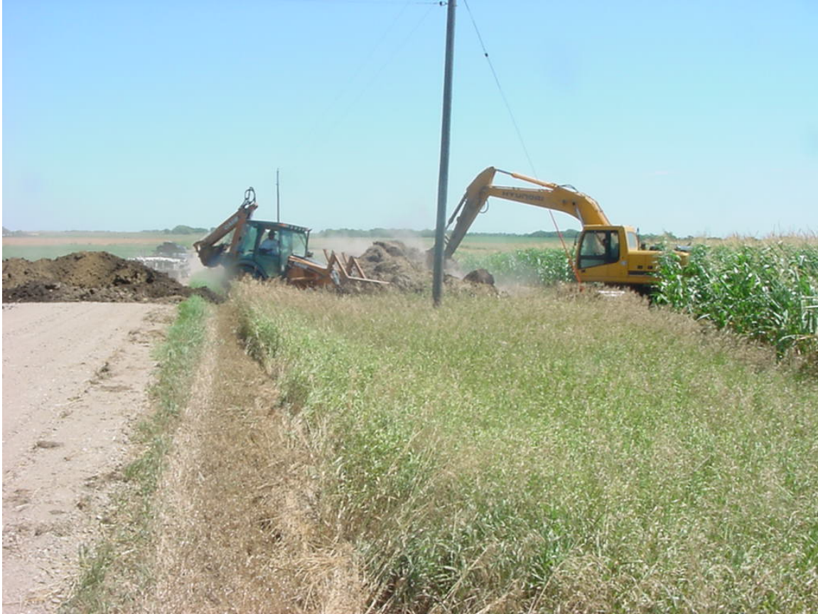
Figure 6. Contractor trenching across road for burial of water pipeline
