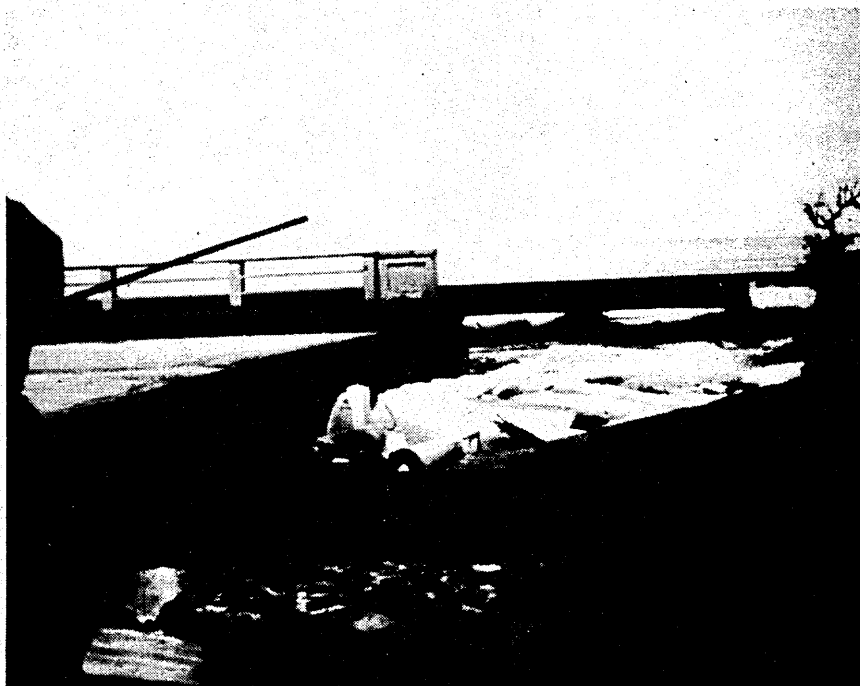
Figure 16. Photograph showing erosion on the east side of Highway 20 Bridge on the inlet-outlet channel (April 10, 1969).
