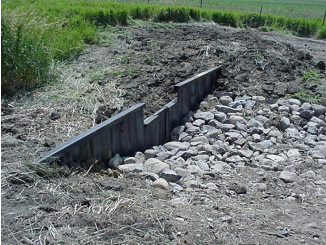
Sheet Pile Structure, Wetland Restoration 2006.
