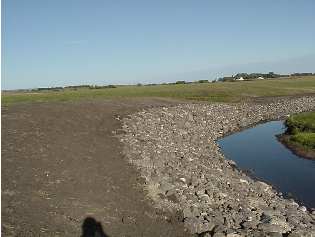
Streambank stabilization completed (Fall 2000).
