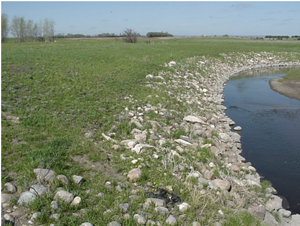
Streambank Stabilization 1.5yr after construction (2002).
