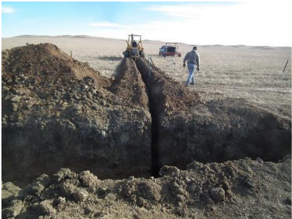
Figure 3-7. Buried Pipeline Installed to Supply Livestock Watering Facilities within the Belle Fourche River Watershed
