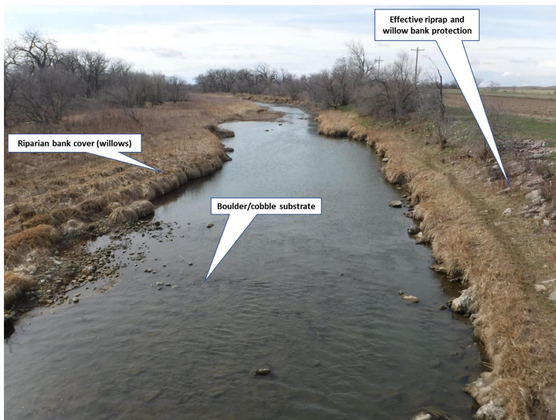
Figure 5-1. Bank Cover, Boulder/Cobble Substrate, and Bank Protection on the Belle Fourche River Above the Fruitdale Road Bridge.
