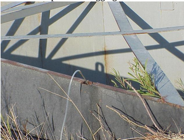
Bubbler tube prone to clogging
