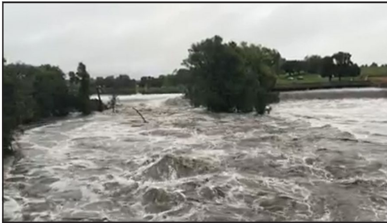
Figure 112. This picture shows the breaching of Platte Lake in September of 2019 after twelve inches of rain. Platte Lake was another WPA era facility on Platte Creek in the project area.
