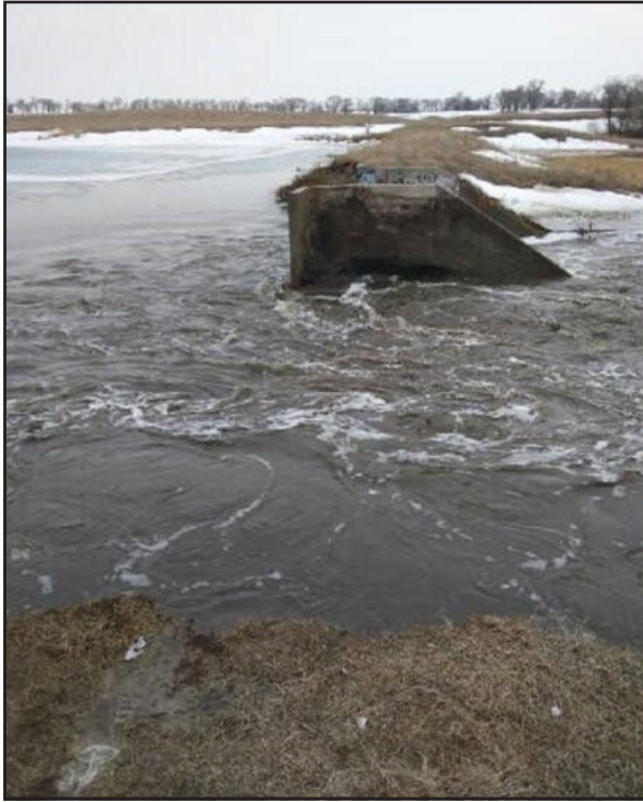
Figure 111. Picture of Hidden Timber Dam breaking as a result of a four-inch rain on frozen ground in April of 2019. This structure was a WPA era dam and was the headwaters for the Keya Paha River in this project area.
